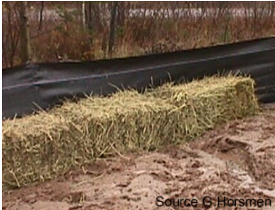
Fig. 3. Hay bales prevent contamination during construction.
